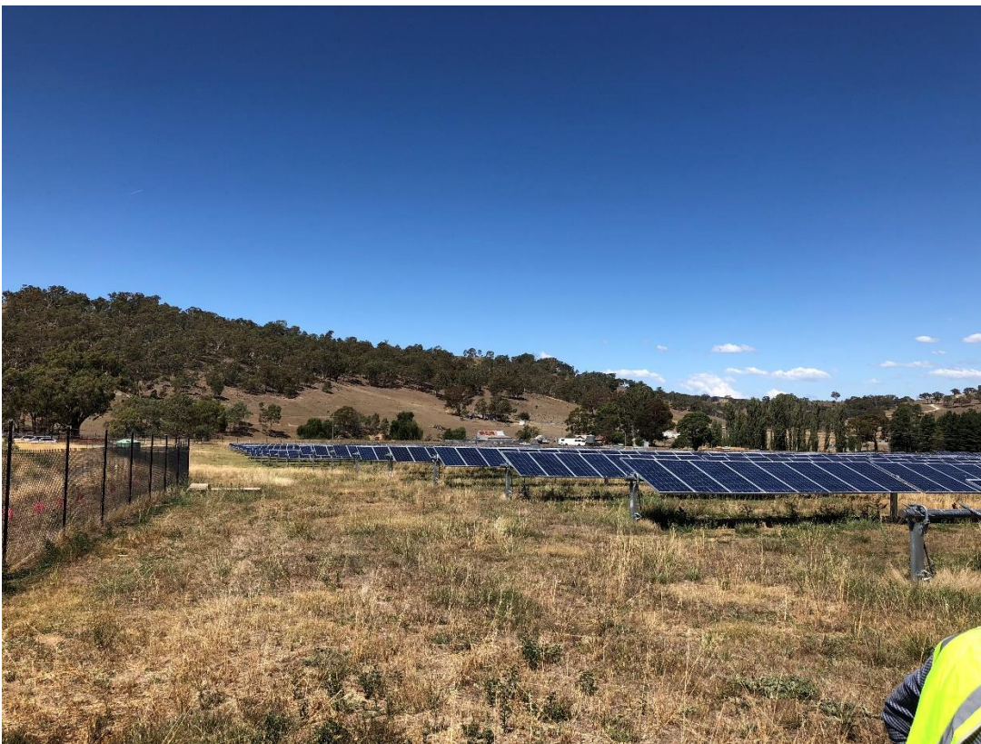
Plate 3: Mount Majura Solar Farm: note provision of stock trough (foreground left) to enable grazing for groundcover management.
